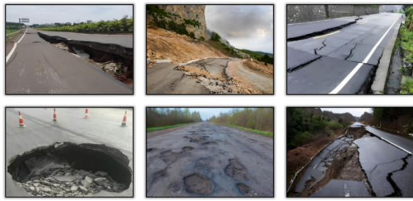
Figure 1: Road diseases caused by loess collapsibility
